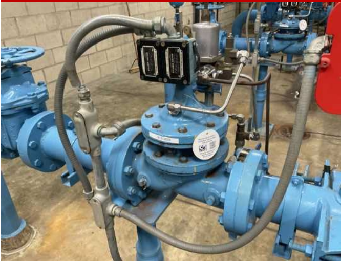
13 - PUMP STATION – MOTORZD CNTRL VALVES
