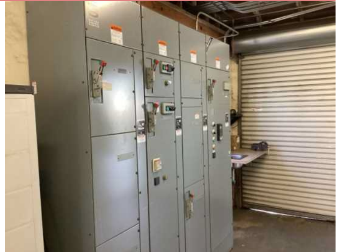
20 - GUNDRY PUMP MOTOR CONTROL CENTER
