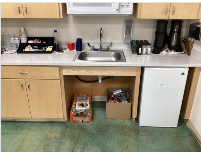
ACCESSIBLE ACCESS UNDER BASE CABINET
