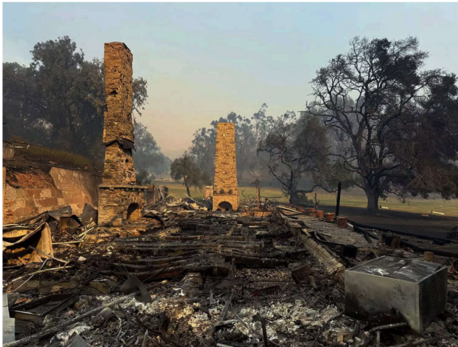
The Palisades fire destroyed Will Rogers' former ranch home at Will Rogers State Historic Park. (California State Parks)
