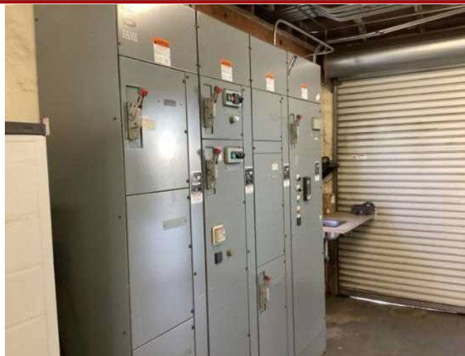
20 - GUNDRY PUMP MOTOR CONTROL CENTER
