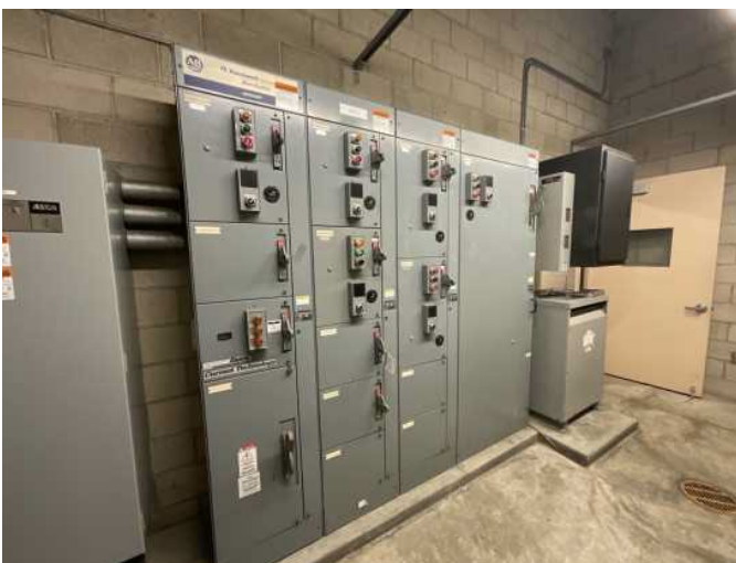
11 - PUMP STATION - MOTOR CONTROL CENTER
