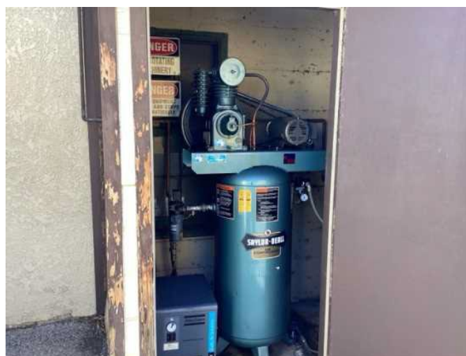
18 - GUNDRY PUMP STATION AIR COMPRESSOR
