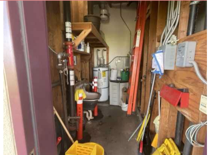
8 - FIRE RISER AND DOMESTIC HOT WATER
