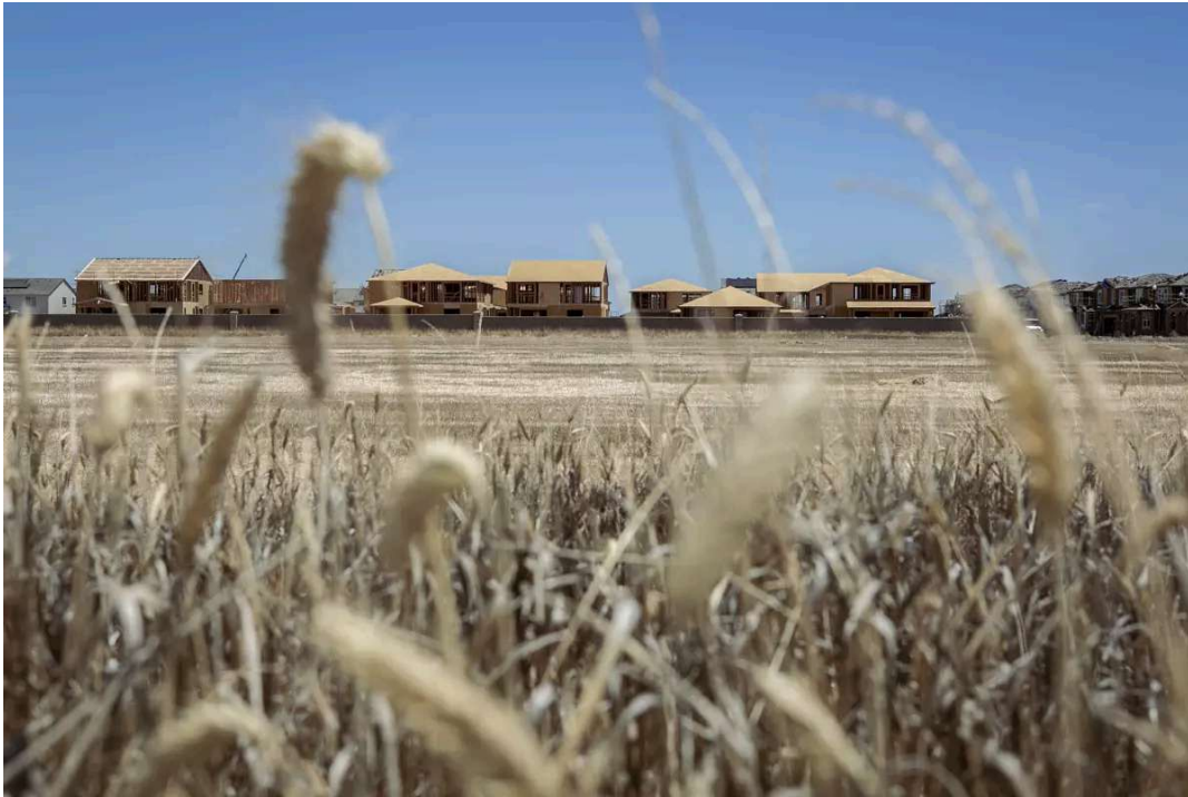
New housing construction in Elk Grove, Calif., in July 2022. (Rahul Lal / CalMatters)
