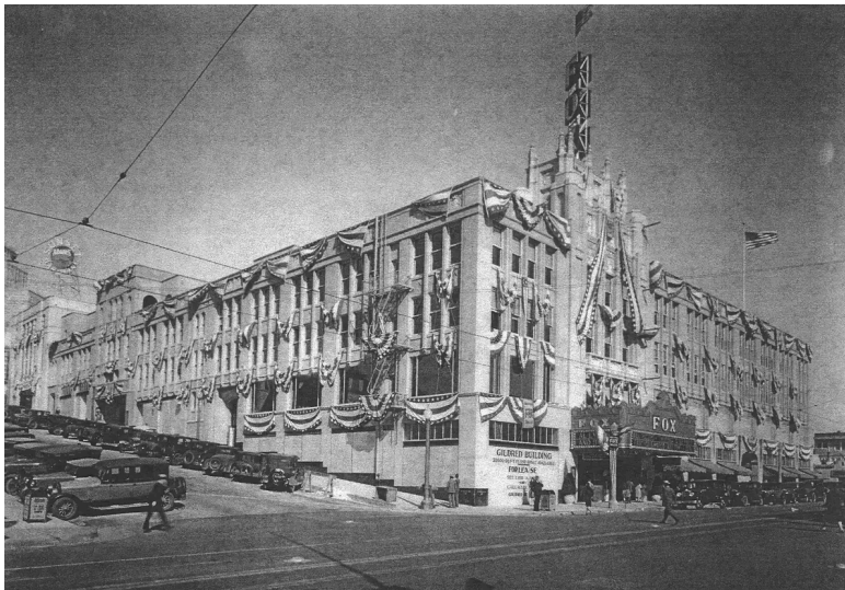
The exteriors of the old Fox Theater were removed in the 1980s. Photo courtesy San Diego Symphony Archives, click to enlarge.
