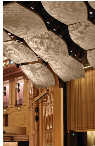
New acoustic reflectors are suspended above the stage. Photo © Richard Barnes
