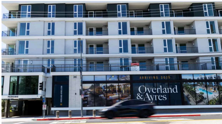
The Overland & Ayres apartments recently completed by GPI Cos. at the site of a former shopping center on the Westside of Los Angeles. (Juliana Yamada / Los Angeles Times)
