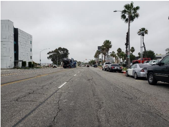
Along Spring Street looking eastbound towards the driveway
