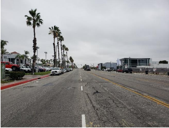
Along Spring Street looking westbound
