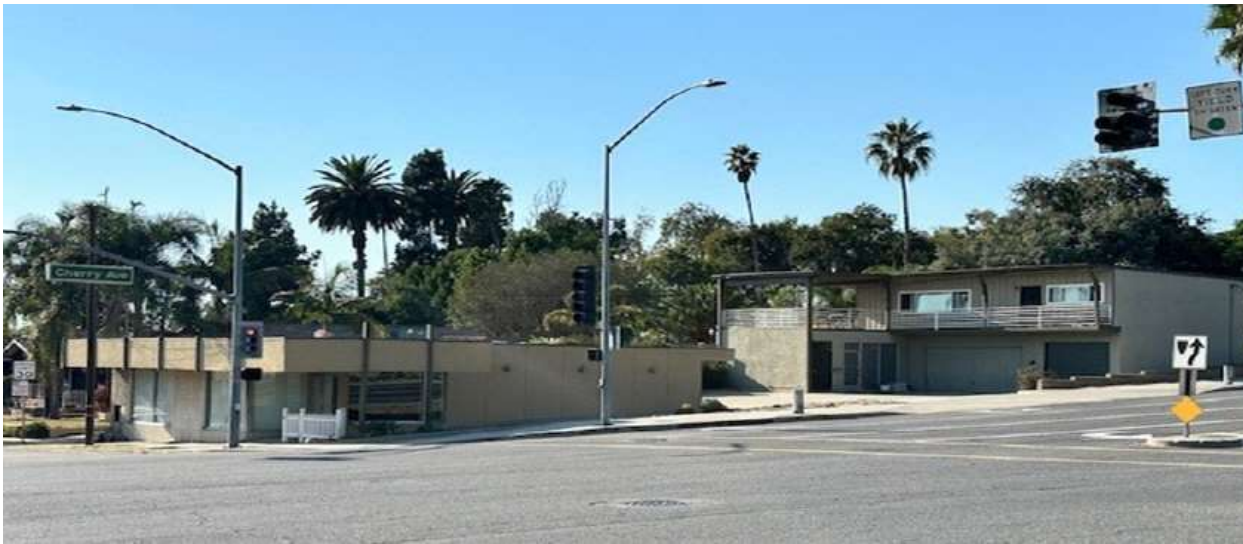
Figure 1: Photograph of the Properties
